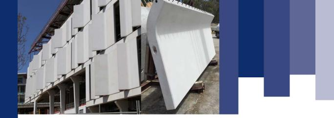
The external façade of the building features curved precast wall panels, manufactured using a full coloured concrete. The panels were then honed to expose the black and white matrix. The curved vertical fins of the precast wall panels help provide shade, thereby reducing cooling costs and results in a building which is industry- leading in its sustainability attributes, achieving a 5-star rating.
