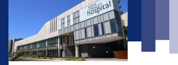
Each of these structures features extensive use of precast, chosen because it offers architectural finishes of various colours and textures that can't be achieved with conventional construction.
